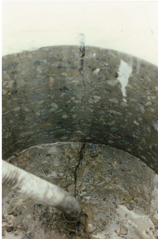
Figure 11: "Sympathetic" crack in CTB below transverse joint crack in PCC in the LDC.
