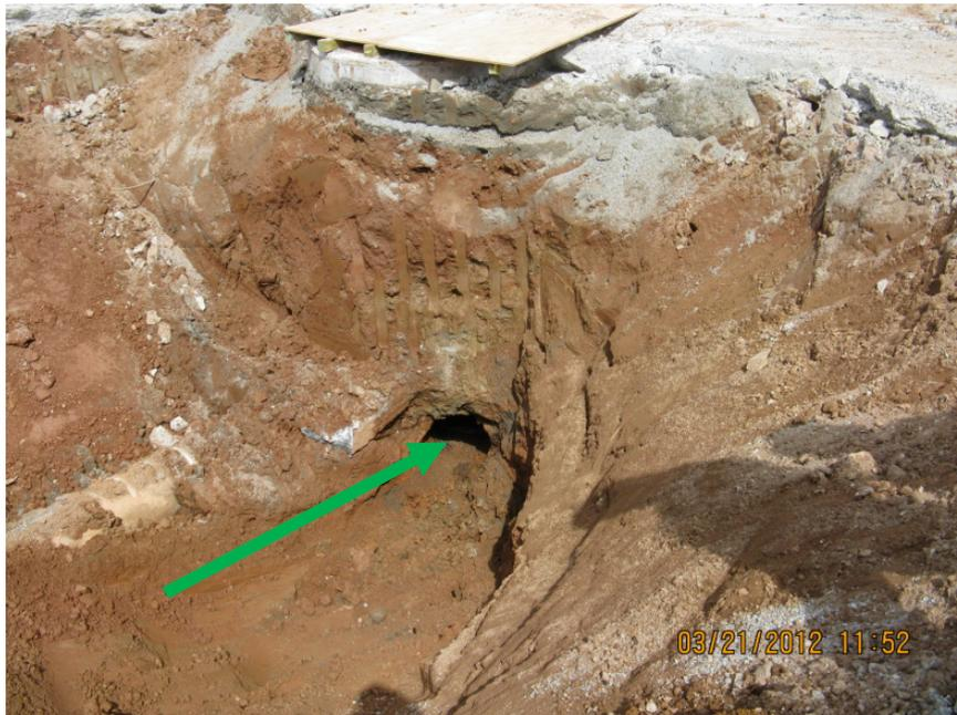
Figure 21: Void and loss of soil in opening in improperly plugged abandoned CMP drain line.
