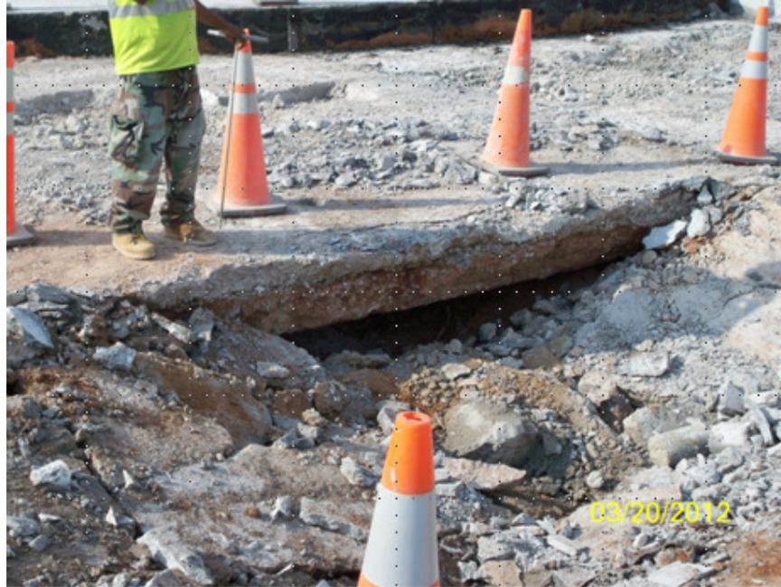
Figure 20: View of void beneath SC and CTB observed during the demolition in the preliminary repair procedures (PCC has been removed).
