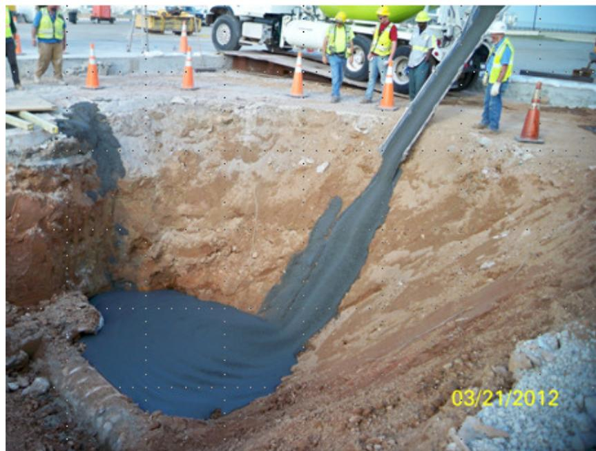
Figure 22: Placement of FCB around the plug in the manhole structure where the CMP entered the manhole.
