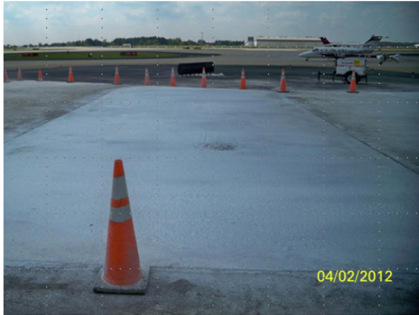
Figure 25: View of completed PCC pavement.
