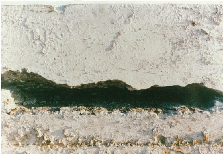
Figure 17: Cracked and sheared zone with pieces removed (Note depth into the PCC).
