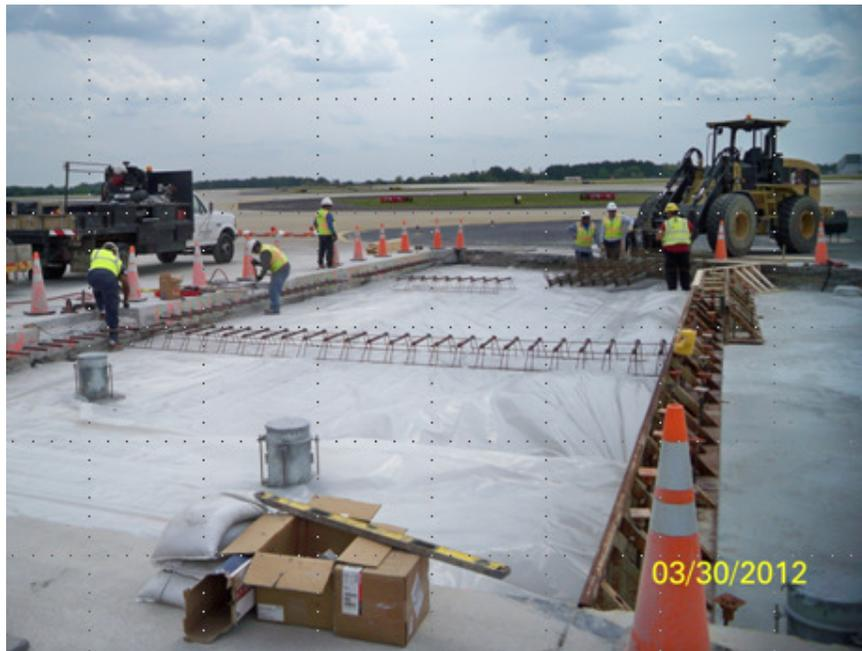
Figure 24: Repair area ready for placement of PCC.
