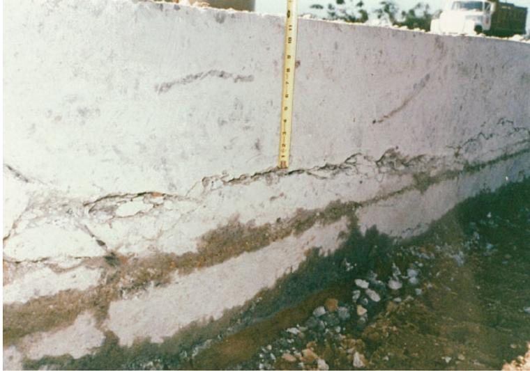
Figure 16: Typical cracked and sheared zone in saw cut face of PCC slab.
