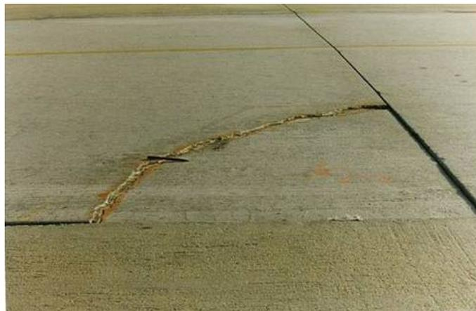
Figure 6: Typical corner crack distress in Taxiway E.
