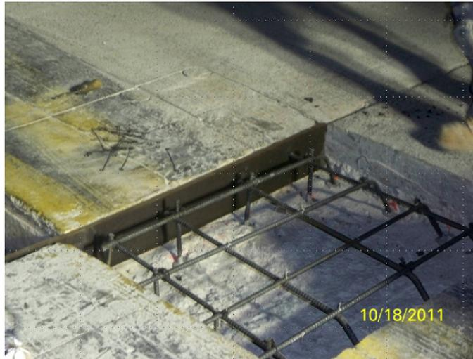
Figure 5: Spall repair showing reinforcing and tie bars to sound concrete below.
