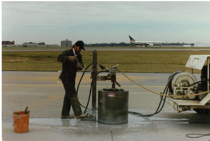
Figure 9: Coring operation for LDC.
