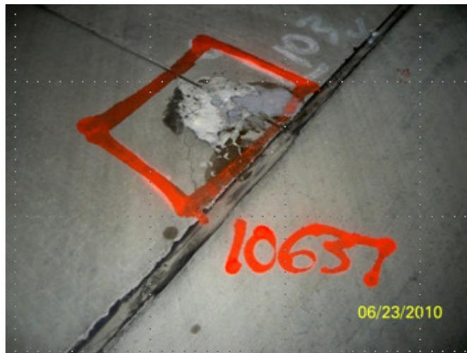
Figure 1: Typical spall distress.
