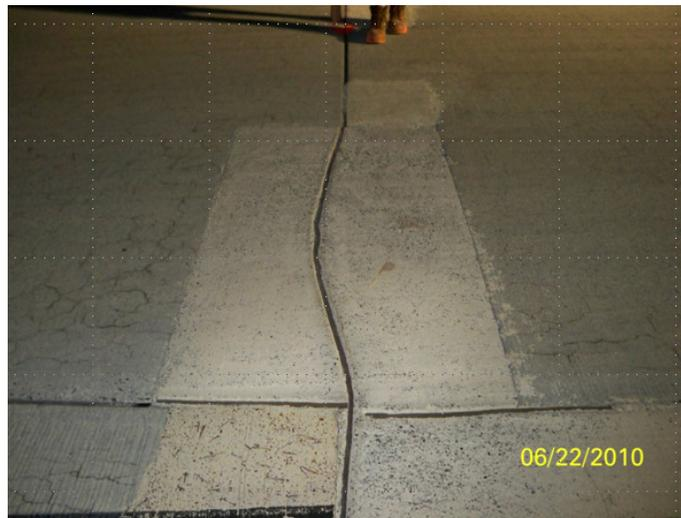
Figure 3: Failure to maintain proper joint alignment and continuity --- future distress.
