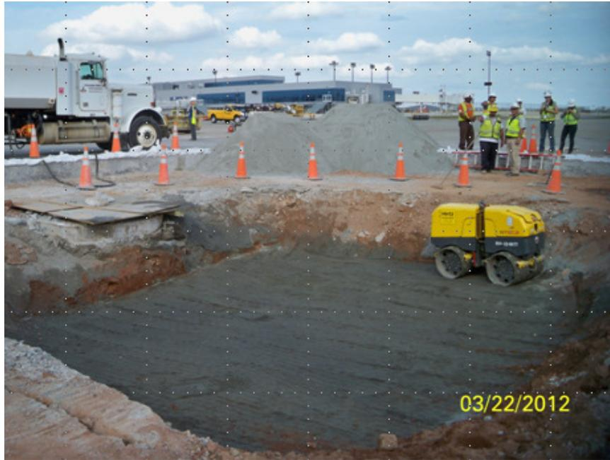
Figure 23: Compaction of M-10 sand above the flowable fill.
