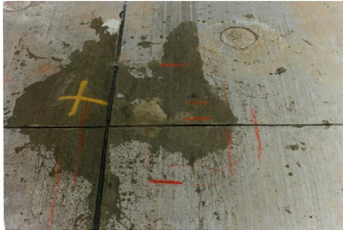
Figure 8: Epoxy used to lock void in place at LDC location (37B).
