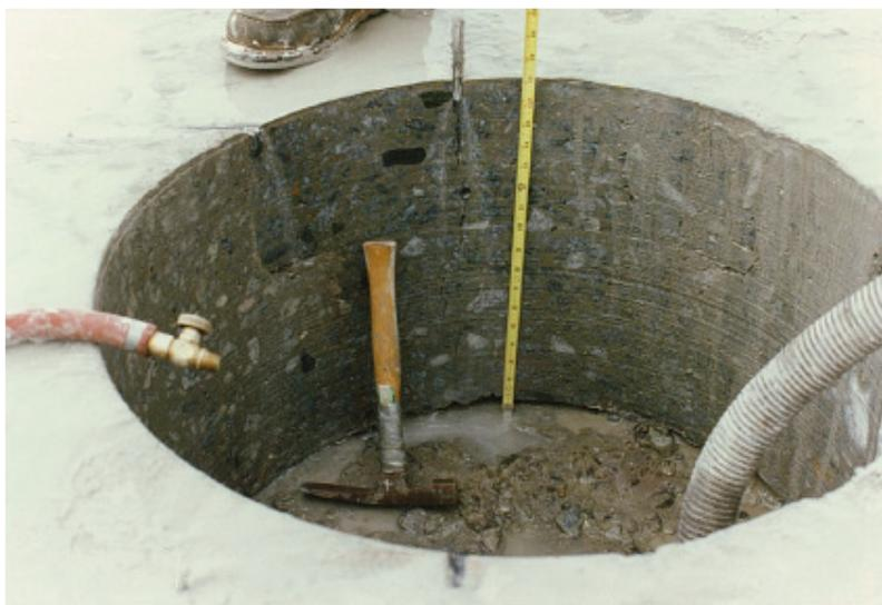
Figure 10: Void between bottom of PCC and CTB in LDC --- void is 19 mm (3/4 inch).
