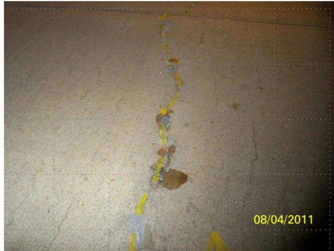
Figure 2: Typical crack routing and sealing distress.
