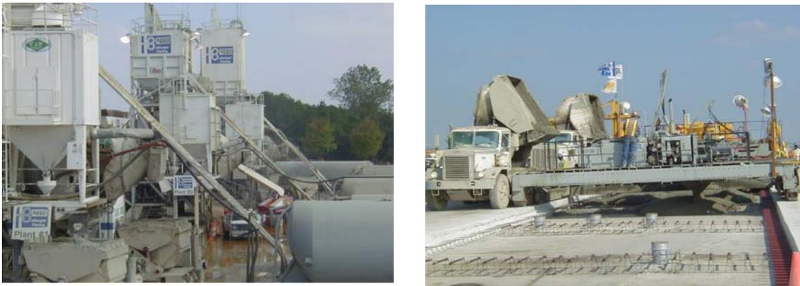
Figure 5 Batching and Placement of Concrete
