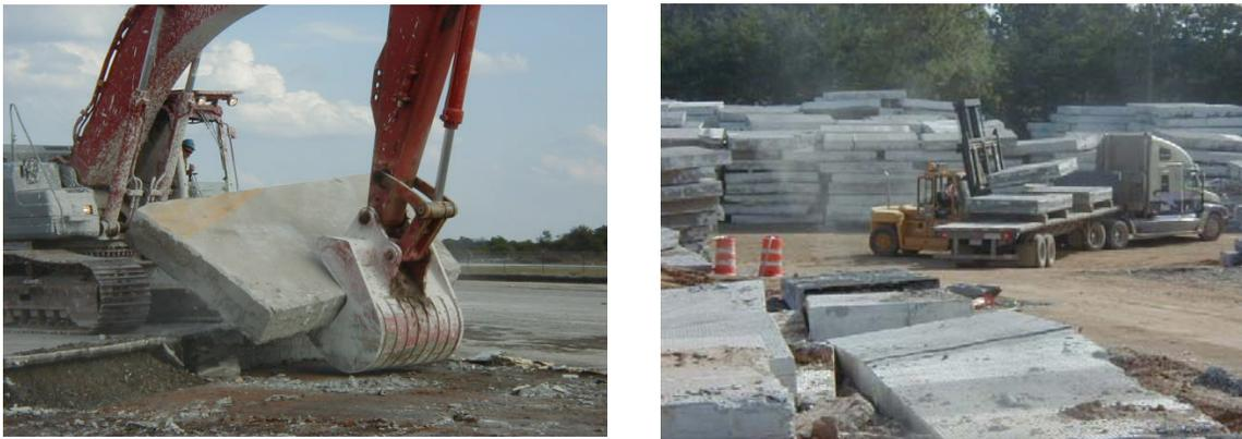
Figure 4 Removal of Existing Pavements
