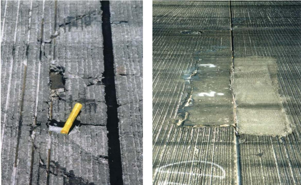
Figure 1 Typical Joint Distress
